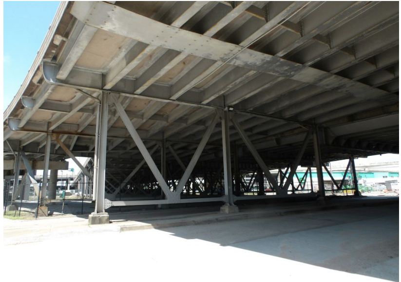
Cross girders/steel pier caps
