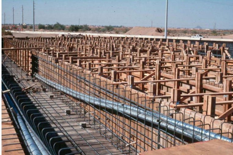
Figure 5-3: Post-tension ducts during construction
