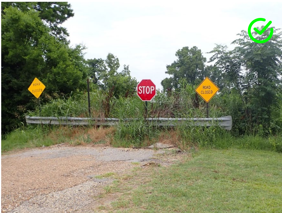
Figure 3-4: Correct closure using guardrail. NOTE: Proper signage should be used
