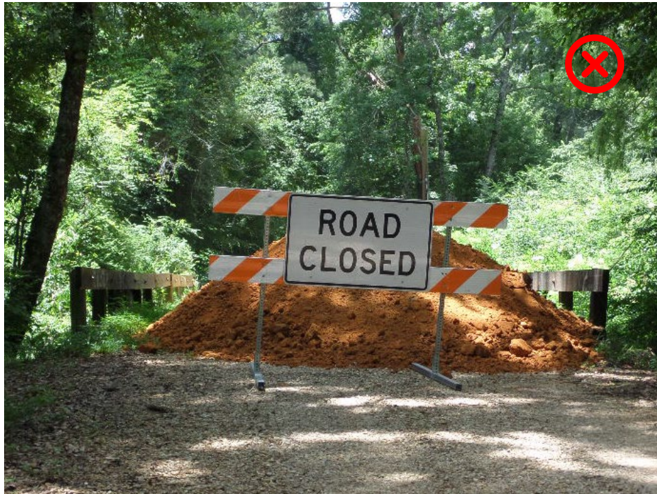
Figure 3-7: Incorrect closure using dirt pile
