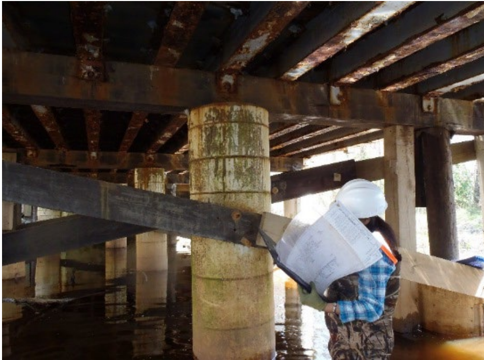
Figure 6-1: "Field" review of bridge inspection
