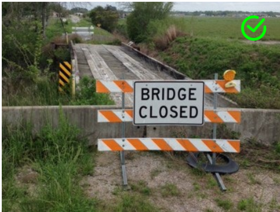
Figure 3-2: Correct closure with Type 3 barricade and concrete barrier
