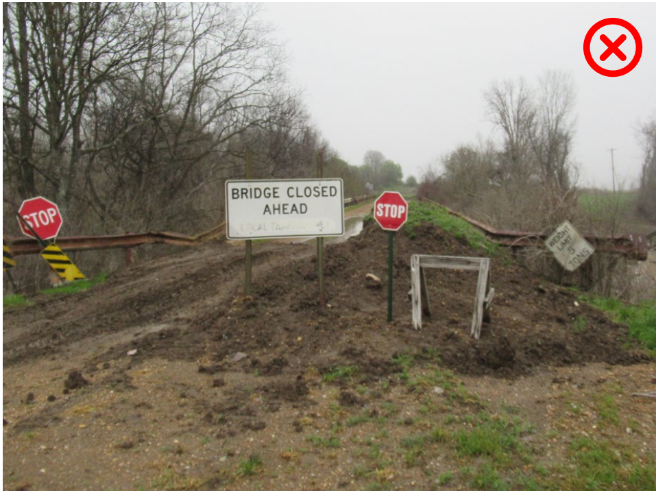
Figure 3-6: Incorrect closure, no positive barrier. NOTE: STOP signs cannot be used for closures.
