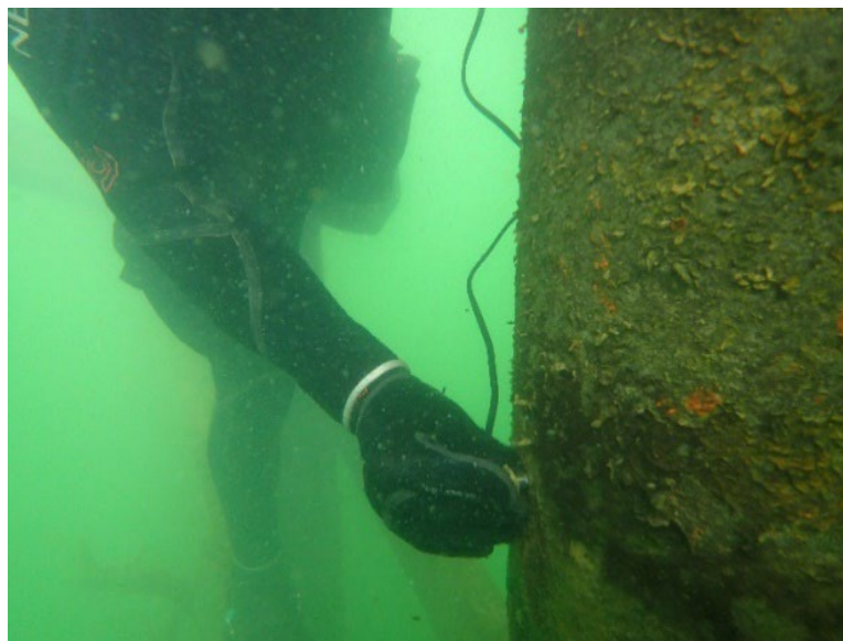
Figure 4-4: UT on steel pile
