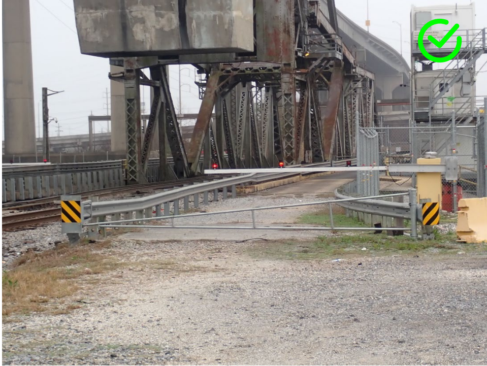
Figure 3-3: Correct closure with a locked gate
