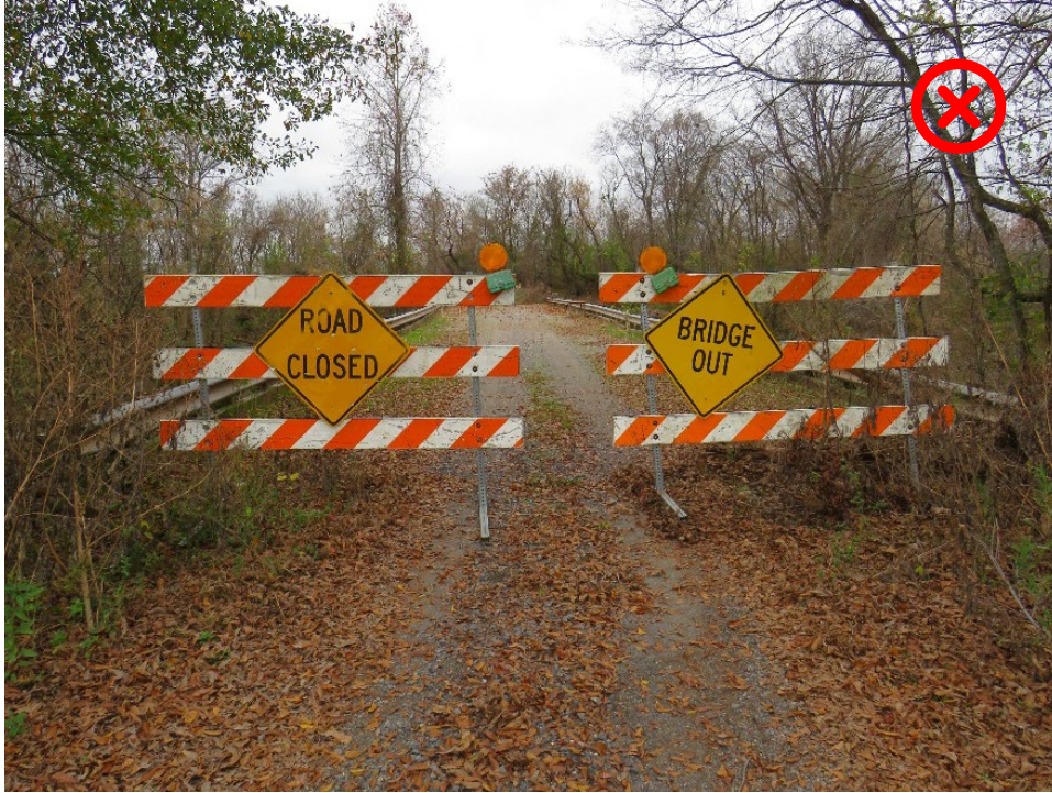
Figure 3-5: Incorrect closure with only Type 3 barricade. NOTE: Signage should not be mixed
