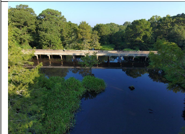
Downstream channel with entire bridge profile shown
