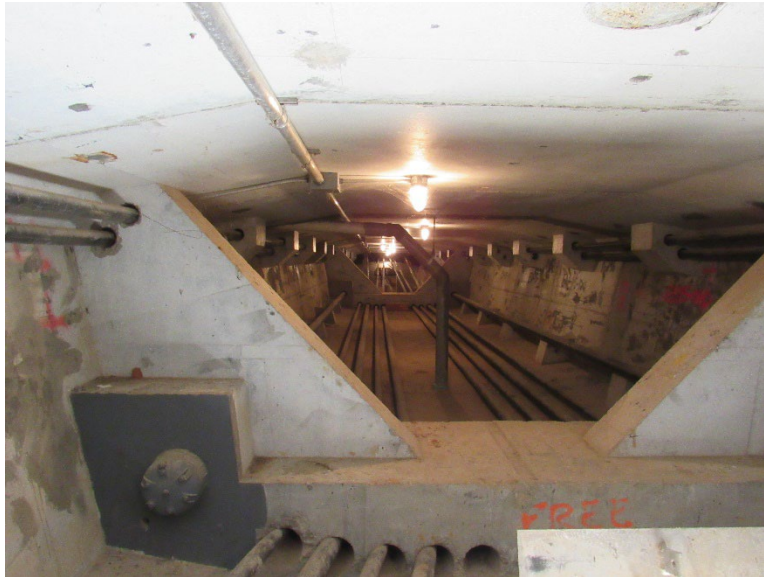
Figure 5-5: Tendon deviation block
