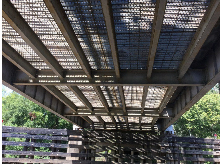
Steel girders and floor beams
