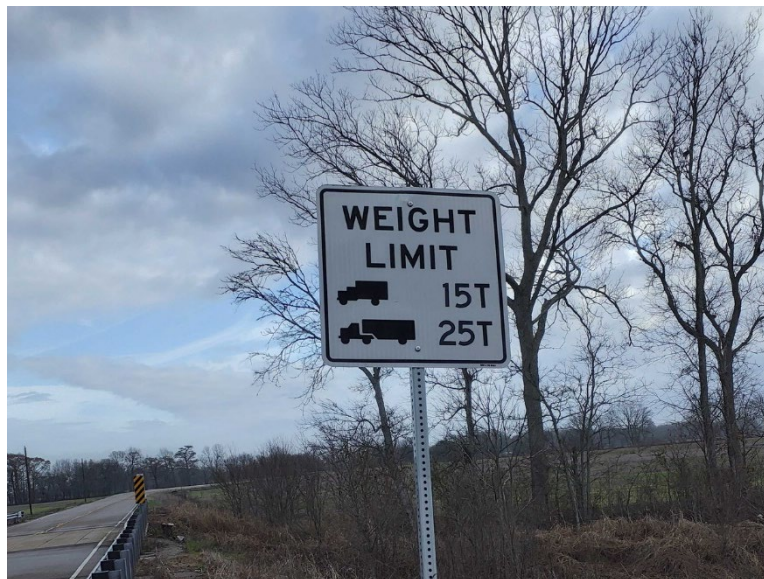
Figure 3-11: Correct weight limit sign
