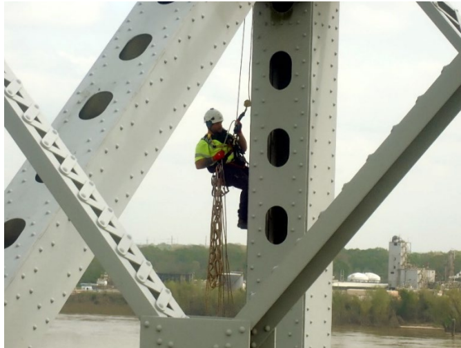
Figure 5-9: Bridge inspection with rope access
