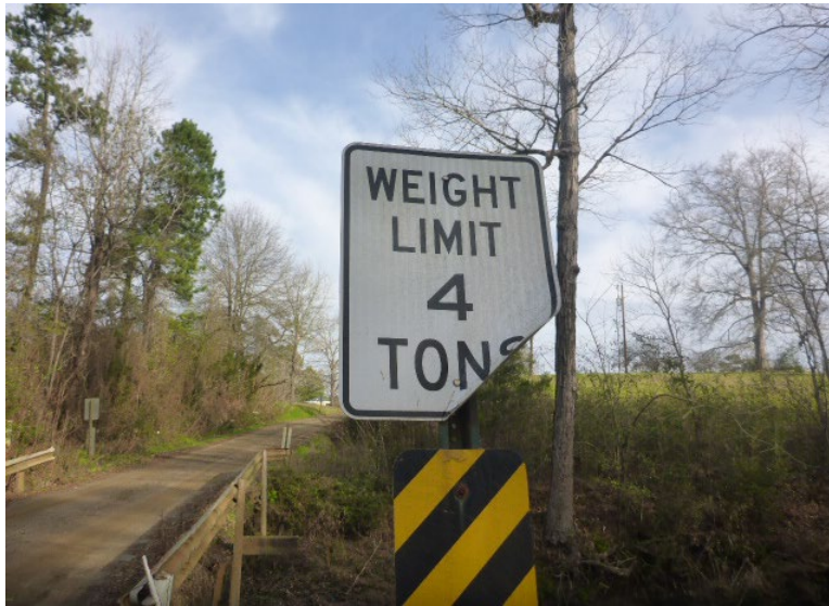
Figure 3-12: Damaged and improper weight limit sign per MUTCD (See Figure 3-8)
