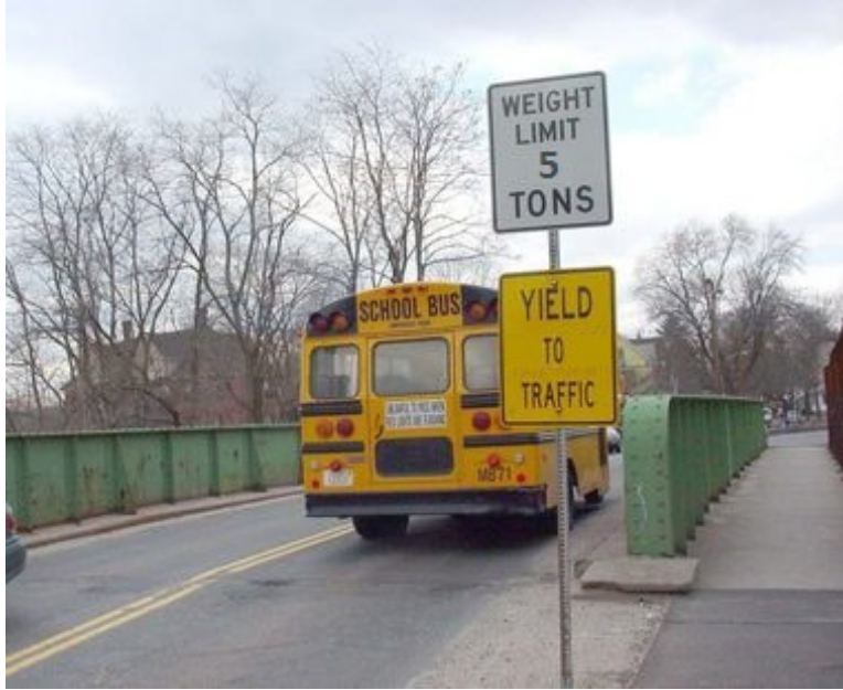
Figure 3-14: School bus violation
