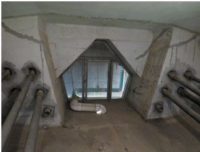
Figure 5-6: Internal diaphragm with tendon anchors
