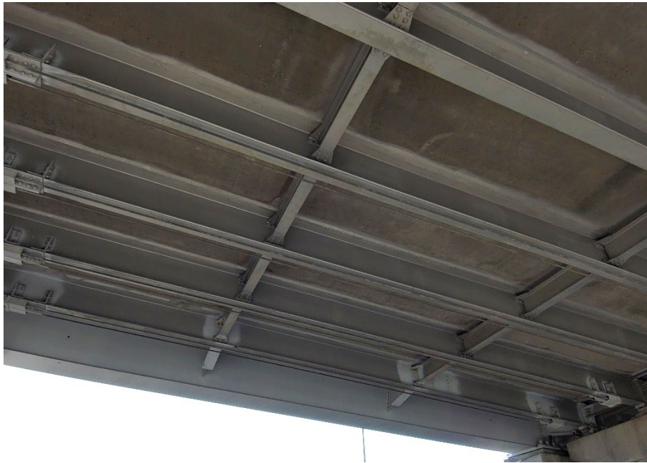
Figure 5-8: External post-tensioned concrete bridge
